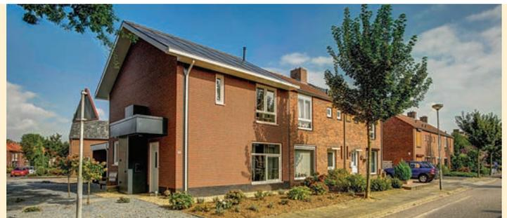
complemented by a services module where renewable energy, grid connection and intelligent management provide heat and power. The envelope and services modules are then delivered to the site to refurbish the existing house, thereby not only insulating the building but providing it with a modern, updated look.
